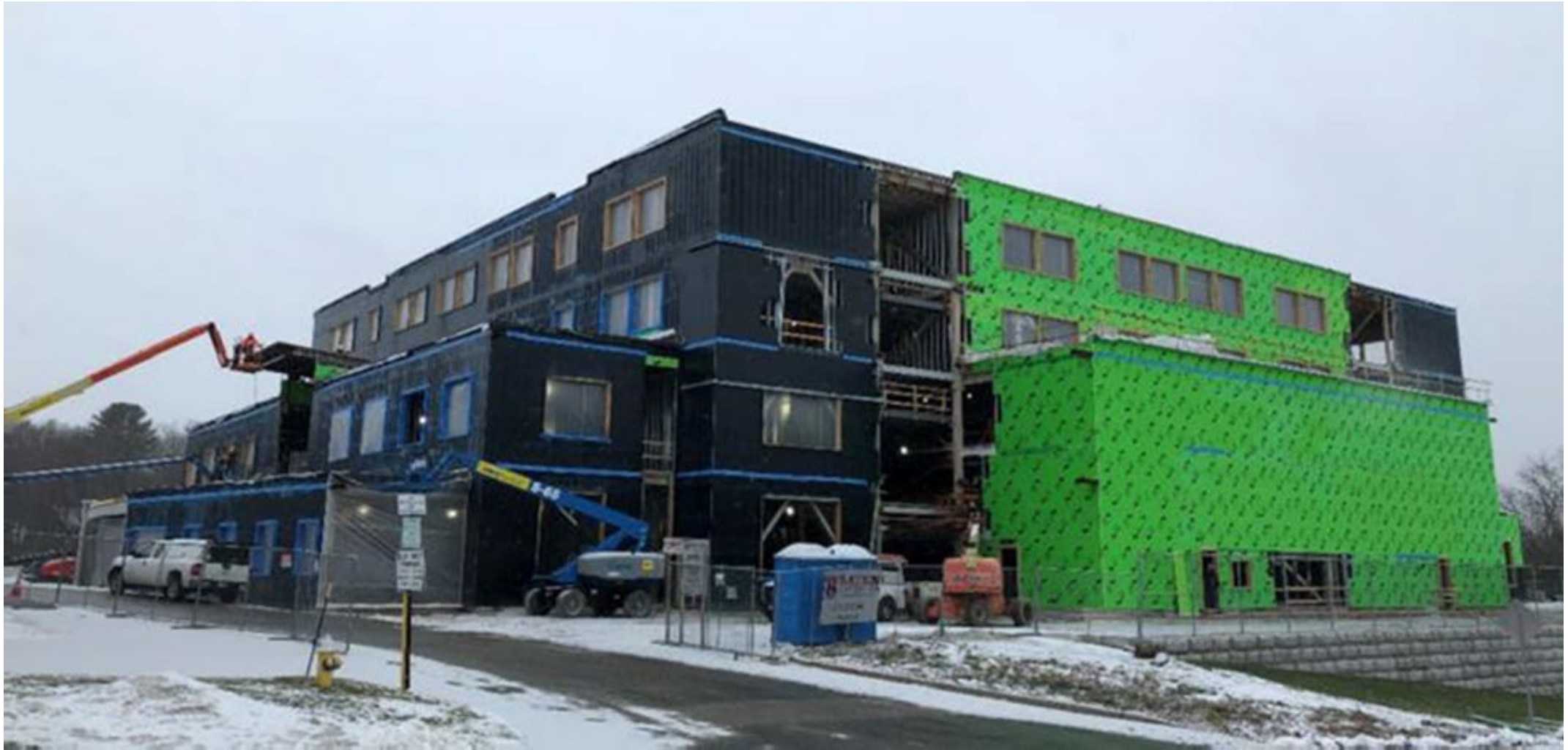
View of South-West Elevation
